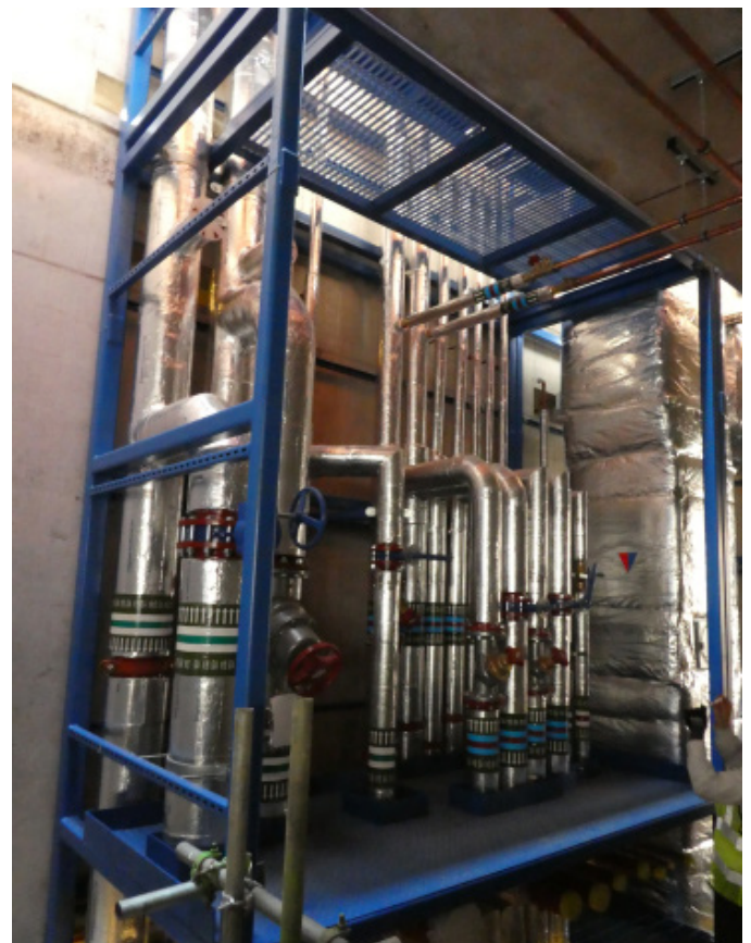
Figure 9: Examples of accessories to facilitate fabrication and installation of prefabricated MEP modules on site (Photograph courtesy of Gripple Limited, Georg Fischer Pte Ltd and Teekay Couplings Ltd)
