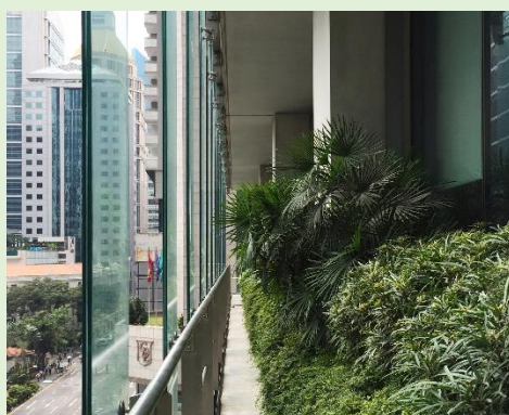
Fig. 4-29 Maintenance access can be designed either in front or behind the verdure
