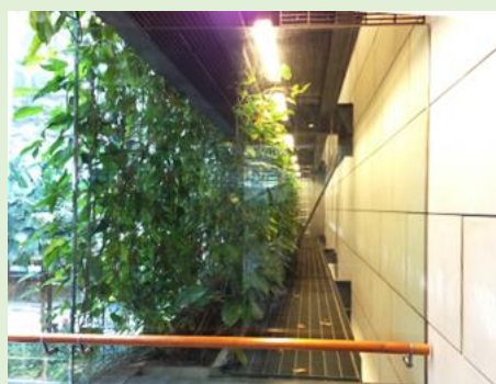
Fig. 4-28 The extent and frequency of maintenance tasks as well as the need for safety features – such as maintenance access, anchorage points and safety lines – should be considered in the façade greenery design
