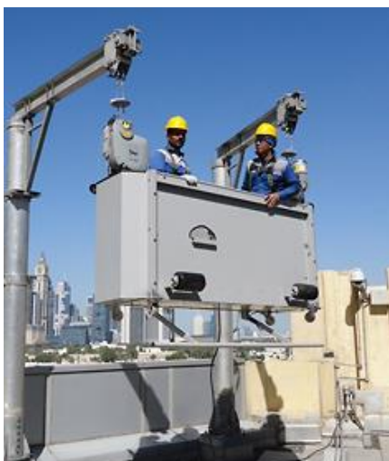
Fig. 3-14 High-profile davits allow the working platform to be launched from the roof top or the ground level
