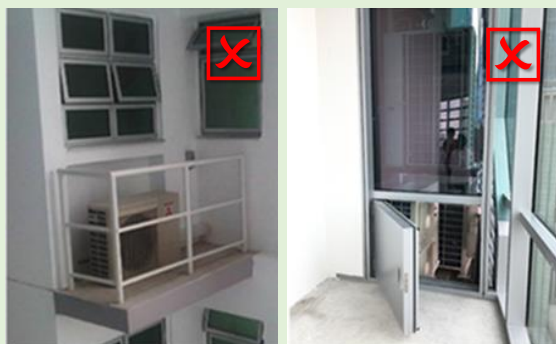
Fig. 4-34 Restricted access openings to AC ledge
