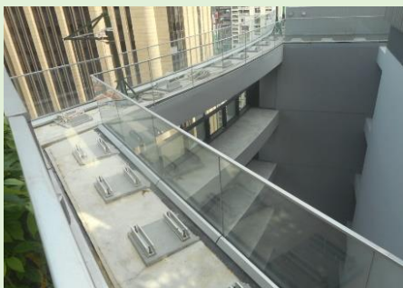
Fig. 4-14 An example of safety barriers
