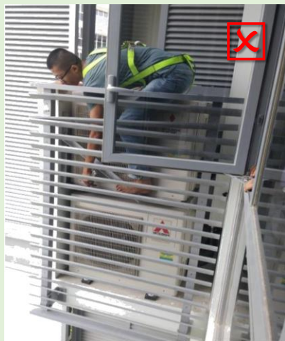
Fig. 4-32 Insufficient working space affects the safety and efficiency of maintenance activities
