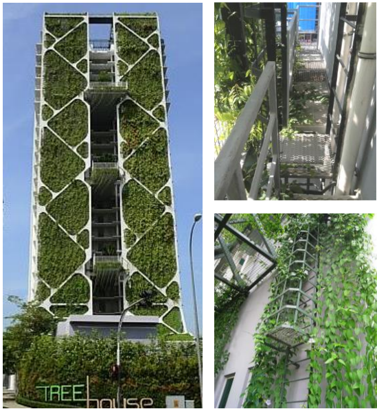
Fig. 2-8 Access ladders and passageways are incorporated in the façade design of Treehouse condominium to facilitate regular maintenance of the façade greenery
