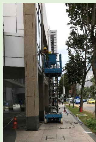
Fig. 4-18 Access and working space for scissor lifts
