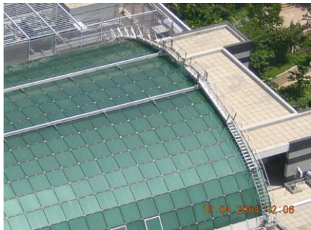
Fig. 3-23 Examples of ladders and gantries used on glass roofs
