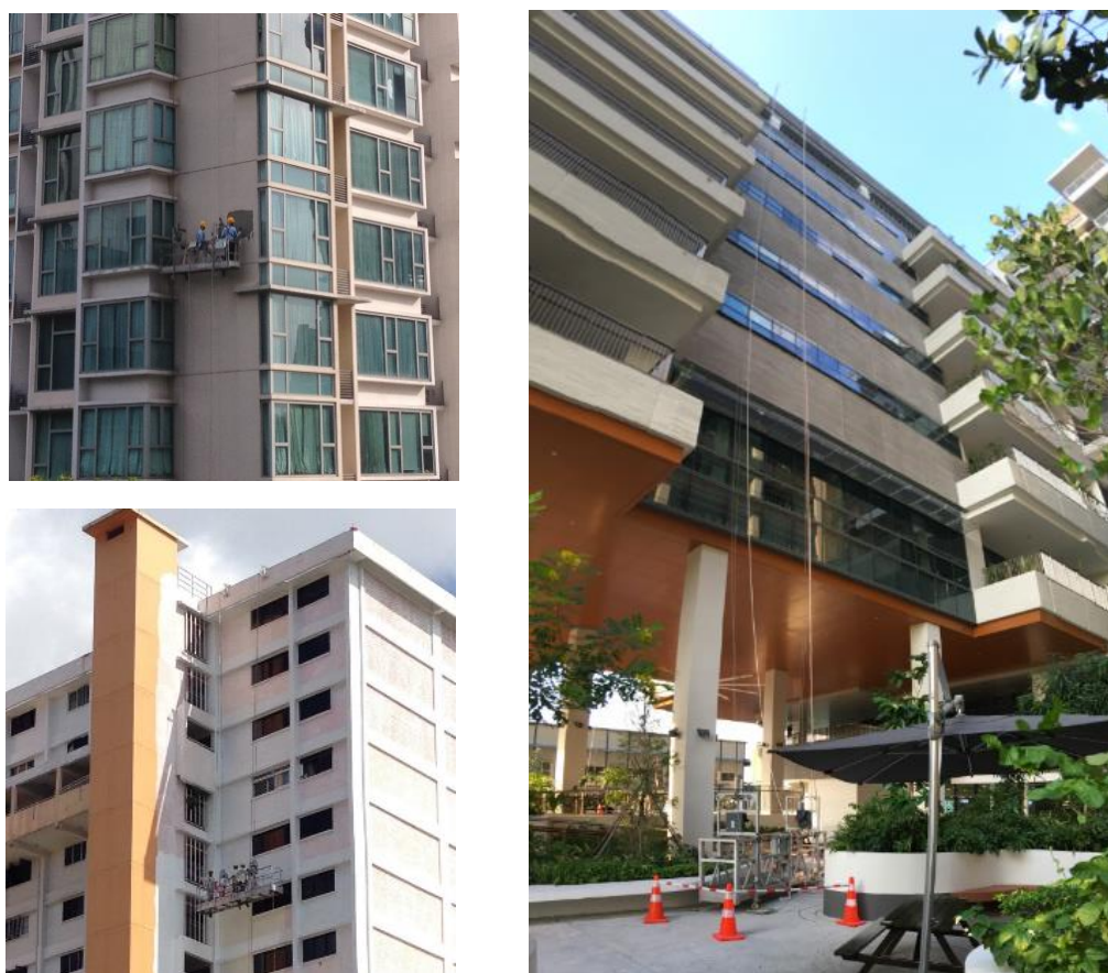
Fig. 3-9 Temporary suspended working platform is a common access system used in various building types
