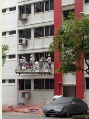
Fig. 4-21 Landing zones should be planned on an unobstructed hard surface
