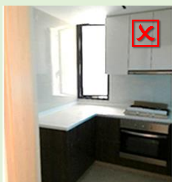
Fig. 4-35 The access opening is poorly located behind the kitchen countertop
