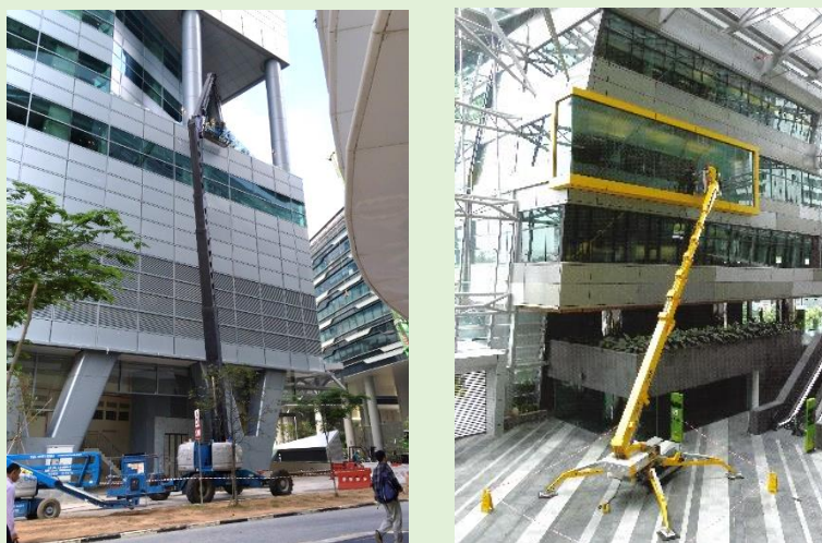
Fig. 4-16 Examples of MEWP in operation
