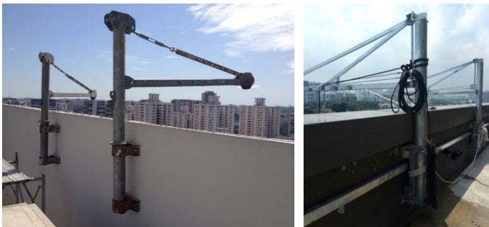
Fig. 3-11 Wall mounted outrigger
