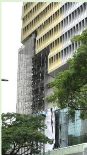
Fig. 4-25 Use of extensive external scaffolding as the primary means of façade access should be avoided
