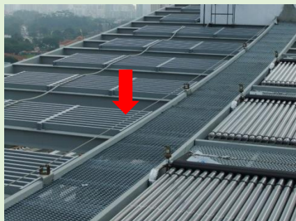
Fig. 4-15 An example of horizontal lifeline
