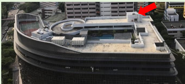
Fig. 4-2 Direct staircase access to the roof
