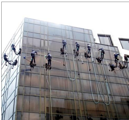
Fig. 1-6 Façade access design should use the most productive means instead of labour-intensive methods
