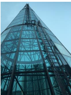
Fig. 3-23 Examples of ladders and gantries used on glass roofs
