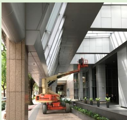
Fig. 4-19 Reach of a MEWP may be affected by overhead structures
