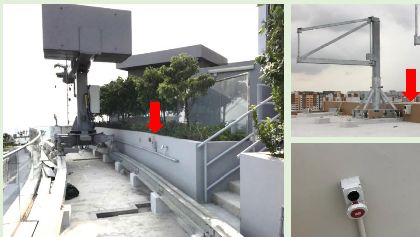
Fig. 4-11 Provision of electrical and water points
