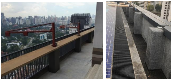
Fig. 3-12 Cast-in outrigger
