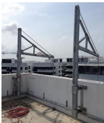
Fig. 3-15 Low-profile davits only allow the working platform to be launched from the ground level. Clear passage around the ground level of the building is needed for rigging and de-rigging procedures
