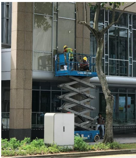
Fig. 3-19 Examples of scissor lifts
