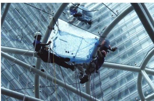
Fig. 3-17 Rope access may not be ideal for more complex tasks such as glass replacement
