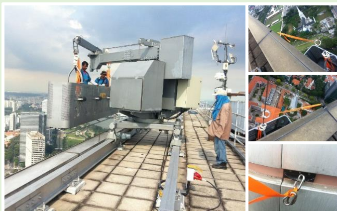
Fig. 4-23 Provision of anti-sway restraints prevent swaying of suspended working platform during windy conditions
