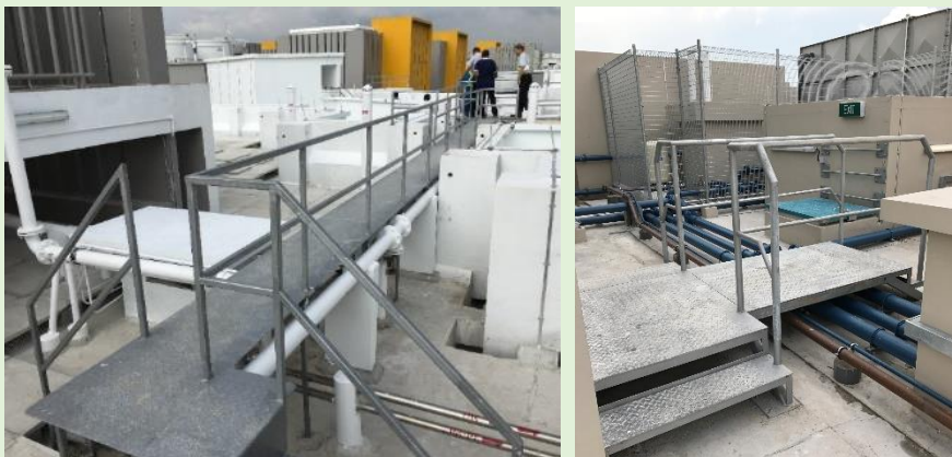
Fig. 4-5 Provision of walk platform over rooftop services
