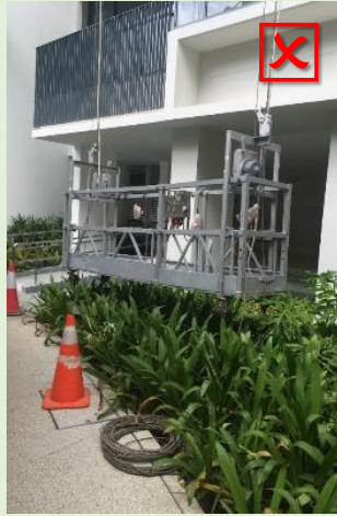
Fig. 4-20 The suspended working platform should not land on PES, landscaped areas or other places that are not suited for landing and rigging operations
