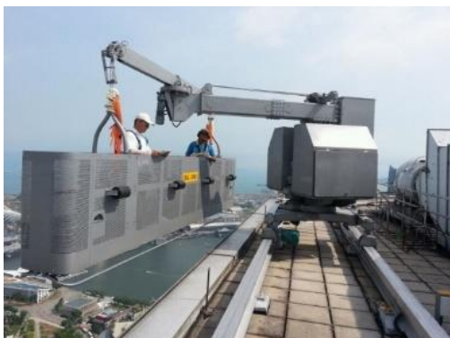
Fig. 3-5 BMU traversing on roof-mounted tracks. Some systems allow the cradle to be detached and use with other rigging system
