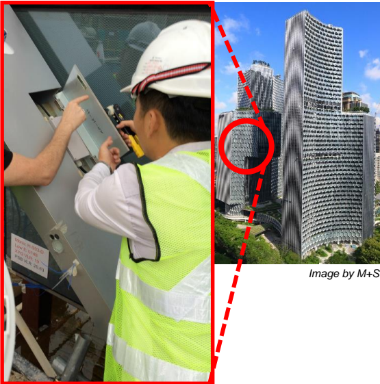
Fig. 2-6 Façade lighting fixtures should be easy to access for maintenance
